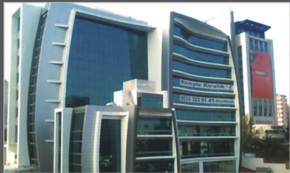
Office building in Istanbul, Turkey.
