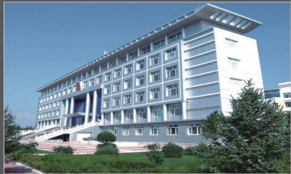
Government building in Inner Mongolia, China.
